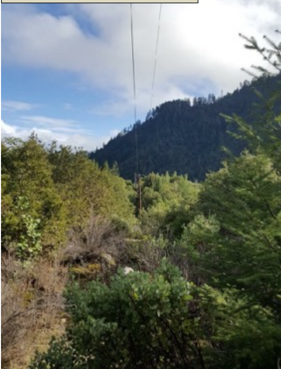
Figure 5.3 Even Maintained Corridors Have Unsafe Levels of Fuels Near Lines
