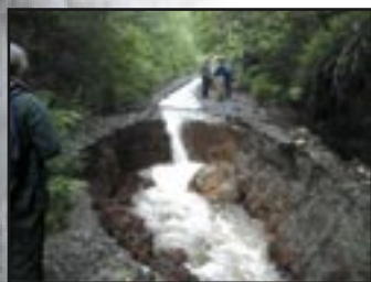
Diverted flow from failed culvert
