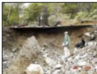
Resulting road damage from failed culvert
