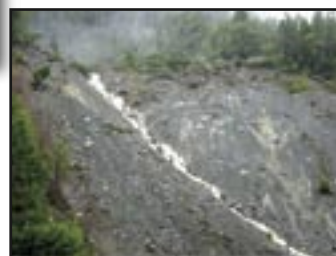
Diverted flow from failed culvert
