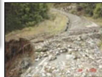
Resulting road damage from failed culvert
