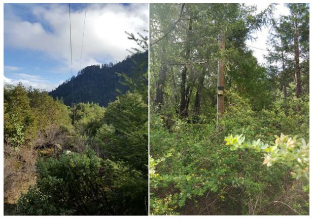
Figure 5 Even Maintained Corridors Have Unsafe Levels of Fuels Near Lines
