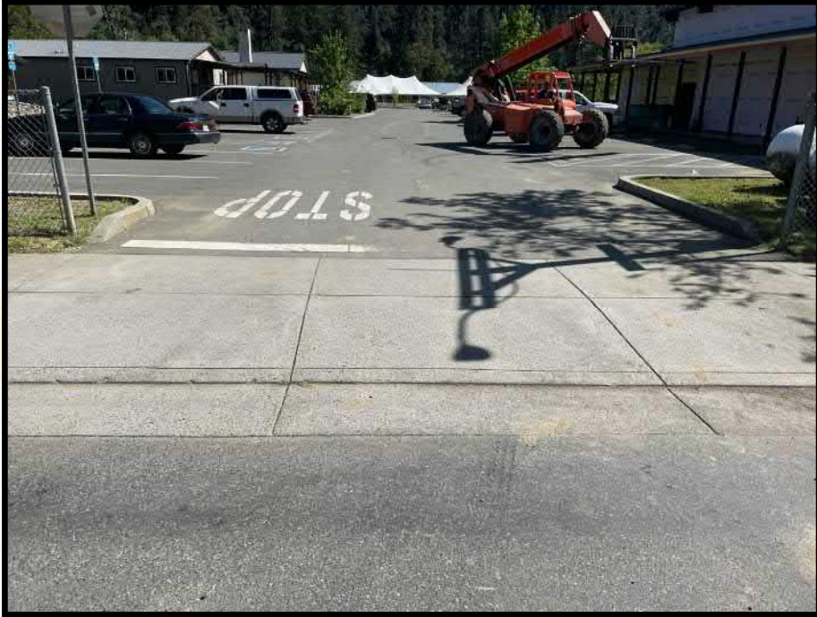
0041_020 7 - Anavkaam Parking Lot
