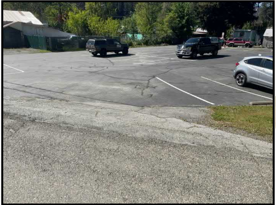
0120_815 1 - Headway Parking Facility
