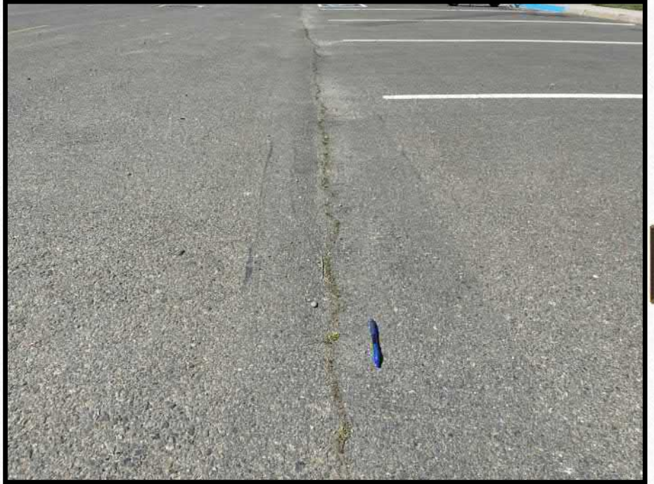
0041_020 6 - Anavkaam Parking Lot
