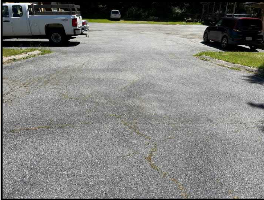
0050_815 3 - Somes Bar Work Center Parking Lot
