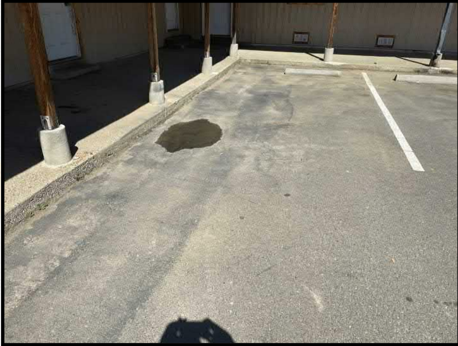
0041_020 5 - Anavkaam Parking Lot
