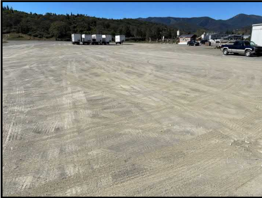
P005_050 3 - Rain Rock Casino Overflow Parking lot
