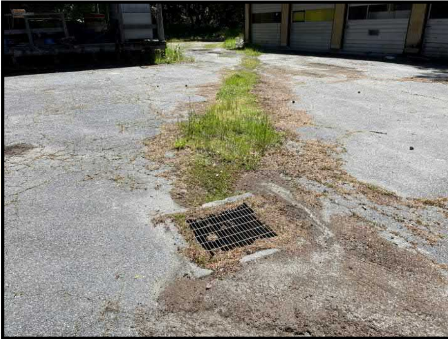
0050_815 5 - Somes Bar Work Center Parking Lot
