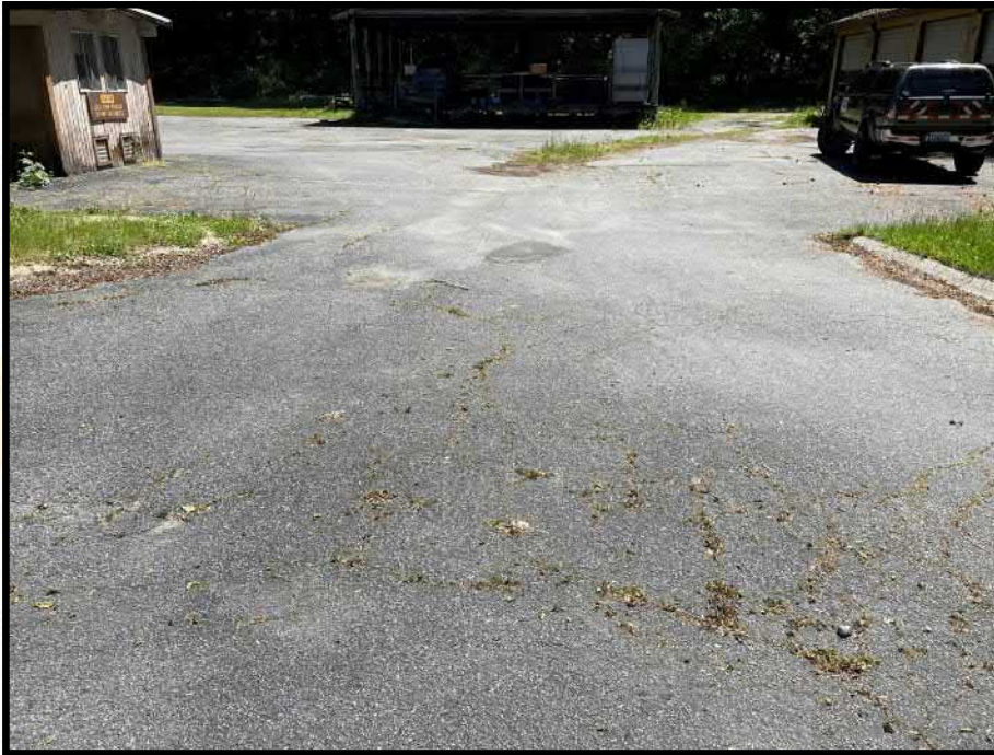
0050_815 1 - Somes Bar Work Center Parking Lot
