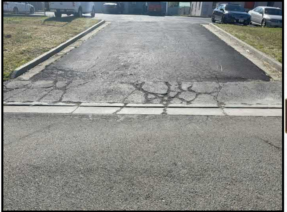
0024_815 1 - KTHA Maintenance Parking Lot
