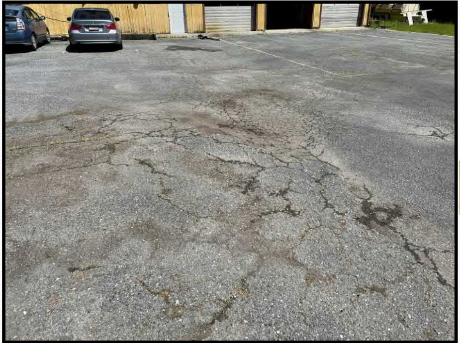
0050_815 2 - Somes Bar Work Center Parking Lot
