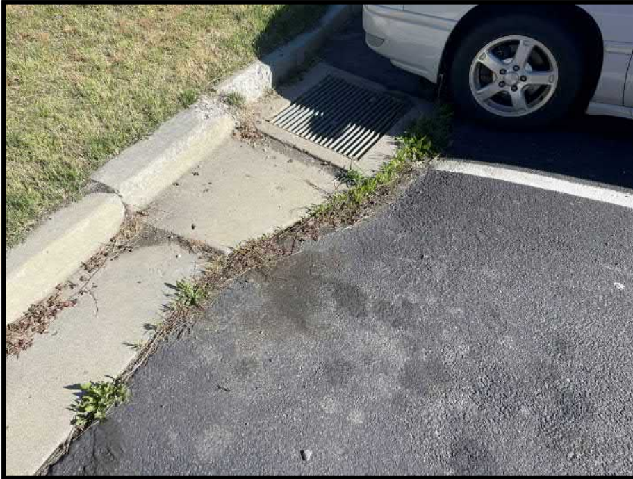
0024_815 4 - KTHA Maintenance Parking Lot
