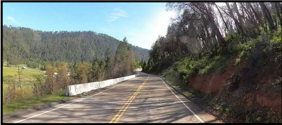
Rt 0111_010(2) - Itroop Rd - Need Object markers on both ends of Concrete Barrier
