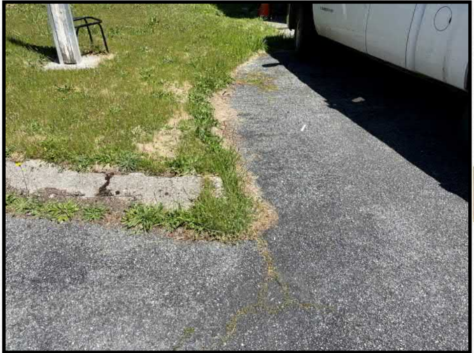
0050_815 4 - Somes Bar Work Center Parking Lot
