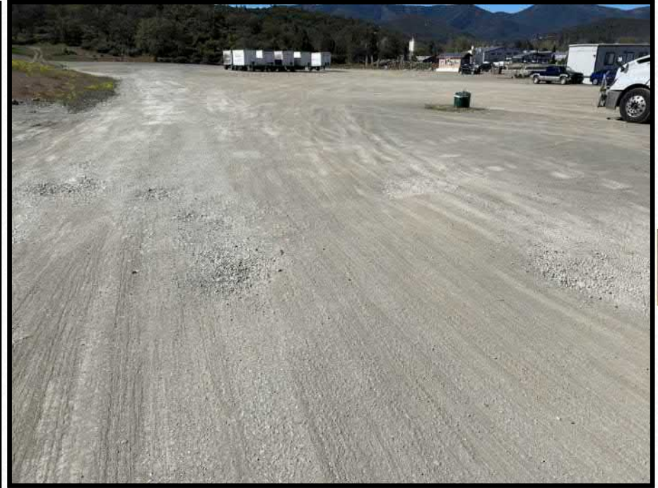
P005_050 2 - Rain Rock Casino Overflow Parking lot
