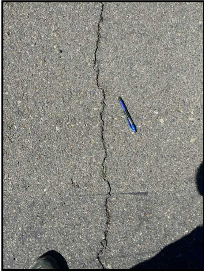
0041_020 1 - Anavkaam Parking Lot
