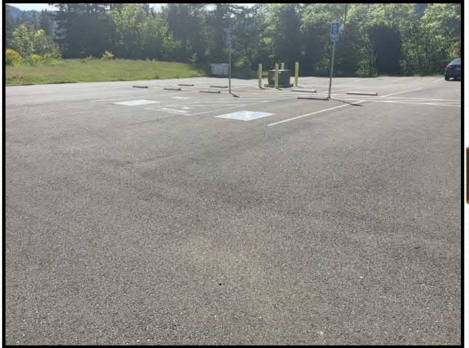
T050_815 3 - Hillside Parking Lot
