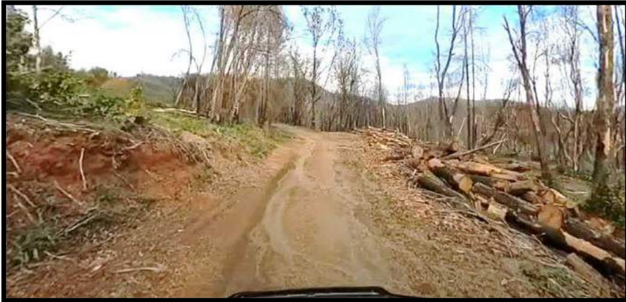
Rt 0111_030(2) - Upper Itroop Rd Erosion issues
