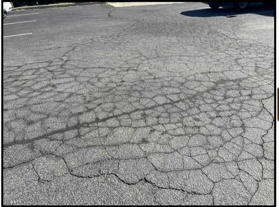
0024_815 5 - KTHA Maintenance Parking Lot
