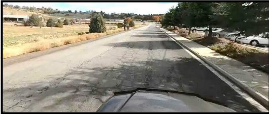
Rt 1014 - Sharps Rd
