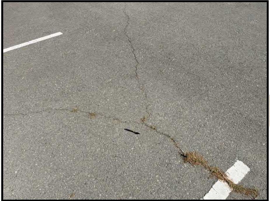
0041_020 2 - Anavkaam Parking Lot
