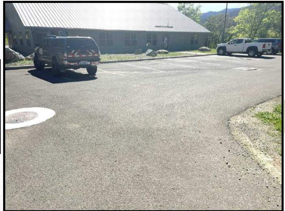
T050_815 1 - Hillside Parking Lot
