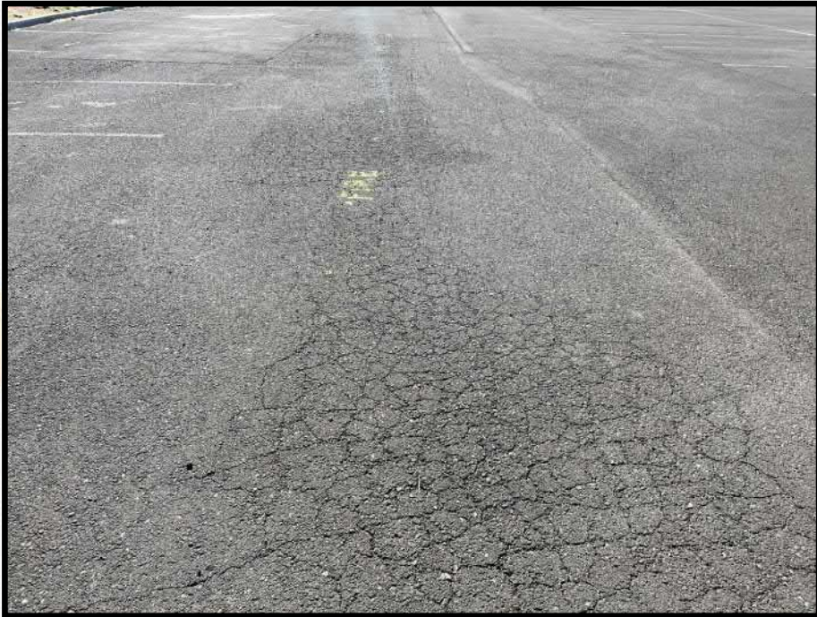
P005_010 3 - Rain Rock Casino Parking lot
