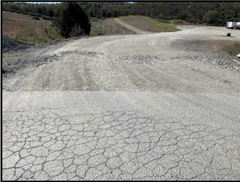
P005_050 1 - Rain Rock Casino Overflow Parking lot
