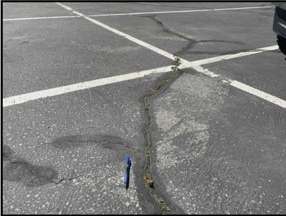
0120_815 2 - Headway Parking Facility
