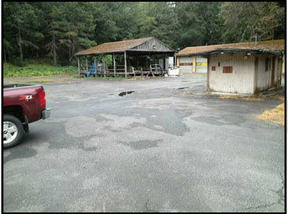
0050_815 - Somes Bar Work Center Parking Lot
