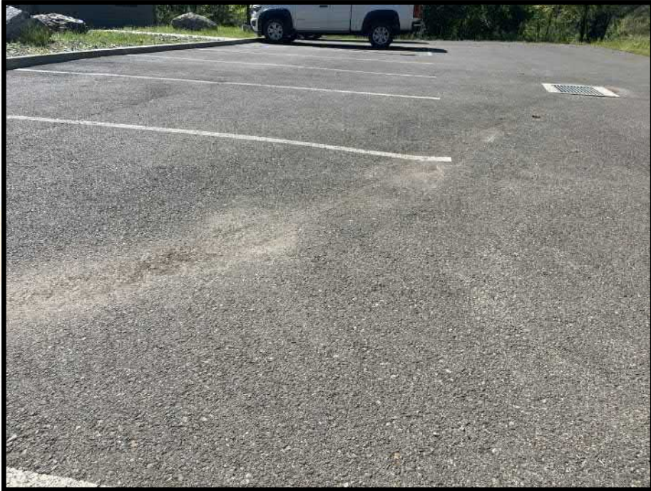
T050_815 2 - Hillside Parking Lot
