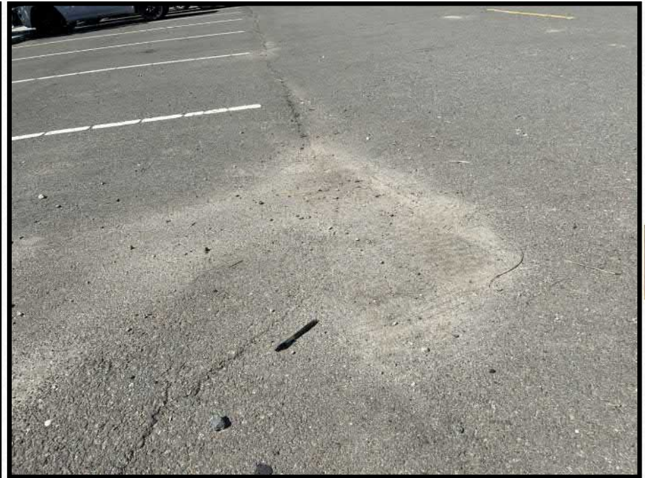
0041_020 4 - Anavkaam Parking Lot
