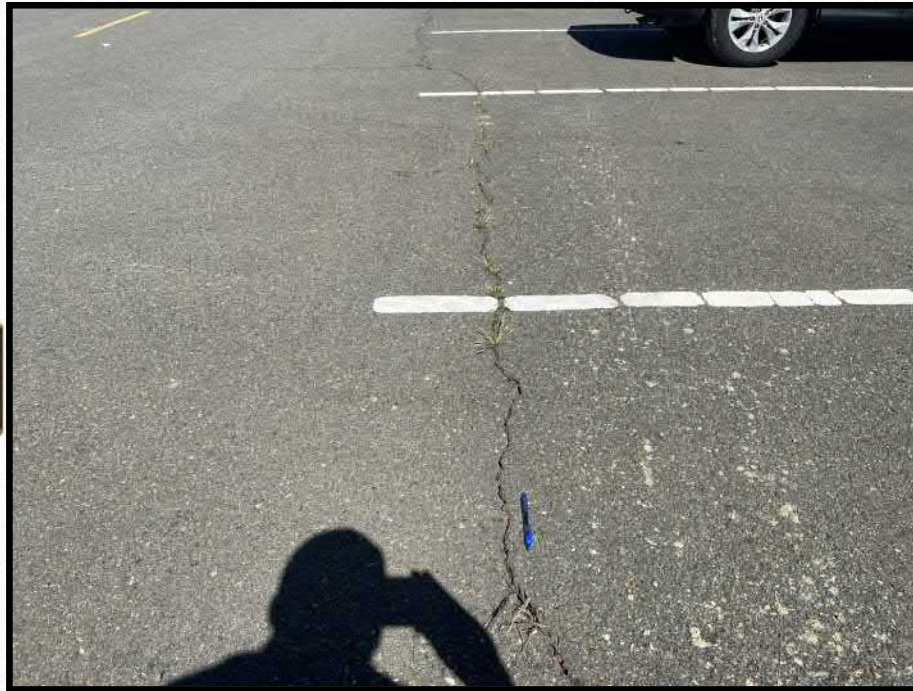
0041_020 3 - Anavkaam Parking Lot
